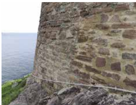
Figure 8 – Tower of Porto: restored surface.
