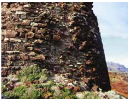
Figure 10 – Tower of Zenòbito: exposed nucleus of the masonry
