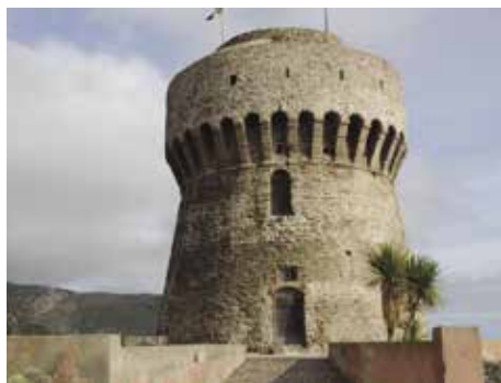
Figure 7 – The tower of Porto, restored.
