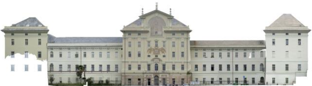
Figure 6. Restitution of the survey of the south façade in 2D digital photogrammetry
