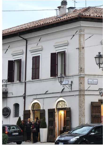
Fig. 3. Norcia. Two-storey buildings, tapered wall thickness, systematic use of tie rods. a) via Cavour, b) piazza Giuseppe Verdi.
