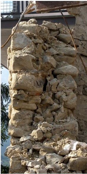
Fig. 11. Poor performance of undressed natural stone buildings in: a) Accumoli, Illica and b) Amatrice, corso Umberto I.
