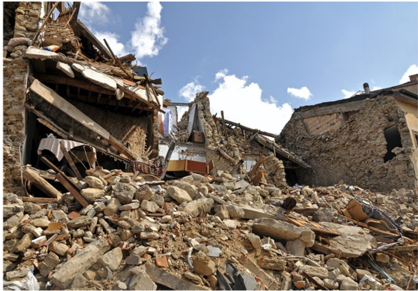
Fig. 11. Poor performance of undressed natural stone buildings in: a) Accumoli, Illica and b) Amatrice, corso Umberto I.
