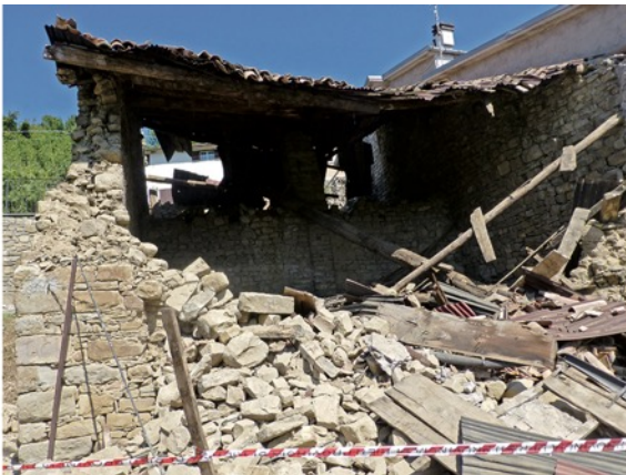
Fig. 12. Masonry disintegration due to poor quality mortar in a reasonably accurate units' assemblage of the external leaf. Amatrice, Cossito: a) Front view, b) detail of masonry on the left-lateral wall.
