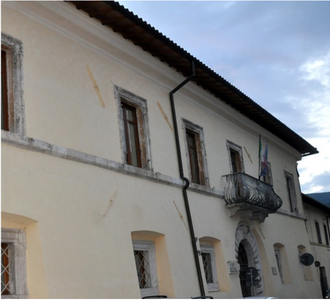
Fig. 3. Norcia. Two-storey buildings, tapered wall thickness, systematic use of tie rods. a) via Cavour, b) piazza Giuseppe Verdi.
