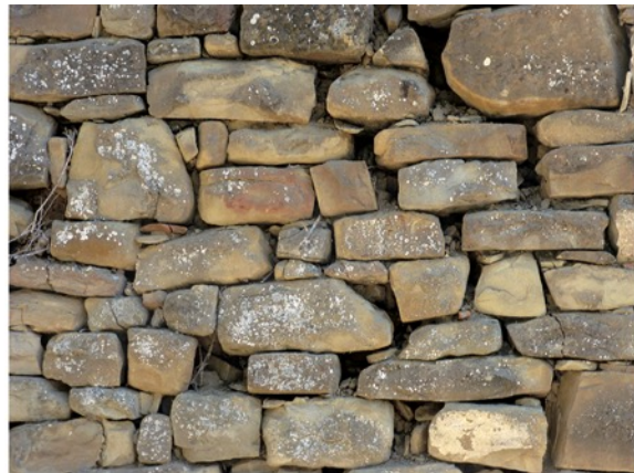
Fig. 12. Masonry disintegration due to poor quality mortar in a reasonably accurate units' assemblage of the external leaf. Amatrice, Cossito: a) Front view, b) detail of masonry on the left-lateral wall.
