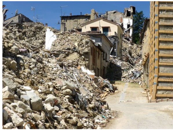
Fig. 10. Damage accumulation in Accumoli, via Tito Vespasiano: a) After August 24 th , b) After October 30 th .
