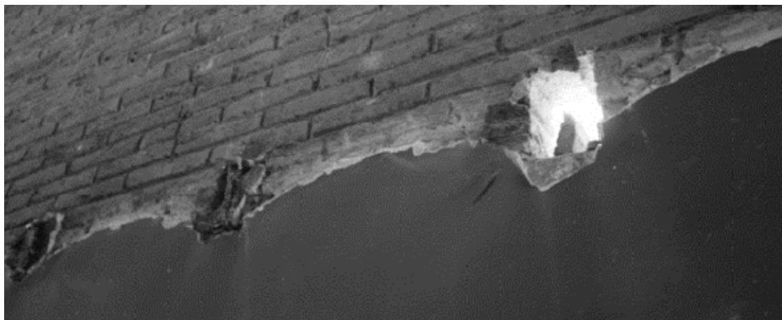
Figure 7. Iron beams (sliced) simply supported on the wall.
