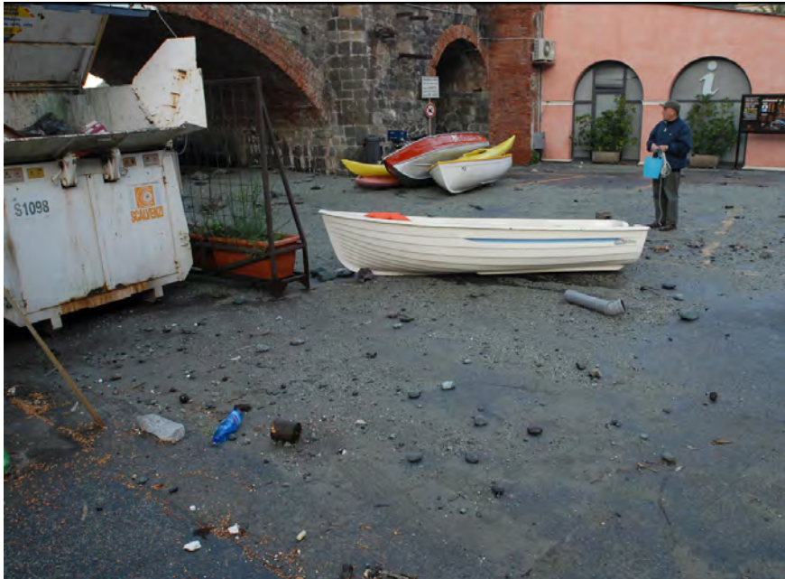
Figure 16: Damage to urban area after 2008 storm surge
