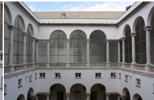
Figure 4 The new design of the Loggia, recurring to high performance glass, allows to close the exhibition space without renouncing to its original visual permeability.
