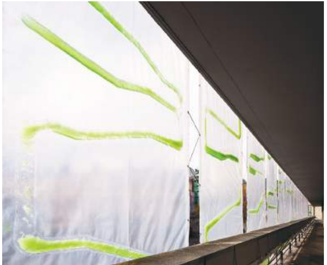
Fig. 8-10 | Photo.Synth.Etica. An urban tent that captures carbon dioxide and releases oxygen thanks to the beneficial acts of micro-algae. A bio-tent envelops the first and second floor of the main facade of the Printworks Building at the Dublin Castle and is composed of 16 modules, each measuring 2 x 7 meters. The proposal suggests the use of cutting-edge technology based on digital and biological intelligence as a potential avenue to addressing the issue of urban design. Architect: ecoLogicStudio (C. Pasquero, M. Poletto); Design Team: K. Alexopoulos, N. Aulitzky, S. Soni, R. Staples, C. Vrantsi, C. W. Yang; Structural Engineering: M. van de Worp – Nous Engineering, USA; Bioplastic Supply and Manufacturing Support: J. Woollard – Polythene, UK; Microalgae Cultures Supply: Dr. Fiona Moejes – Bantry Marine Research Station, Ireland (photos by NAARO).
