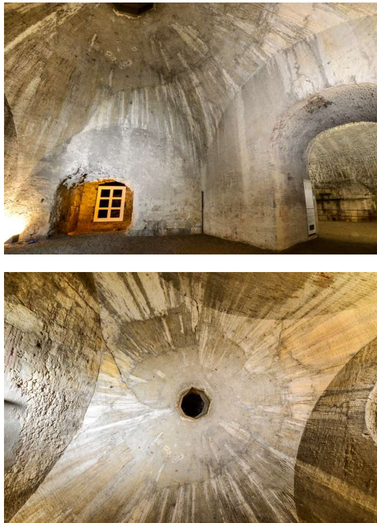
Fig. 1. Sail vault in the Cavaniglia bastion of Fortezza Vecchia: the intrados spherical surface with pendentives ( above ); the octagonal oculus and radial brick bonds ( below ).
