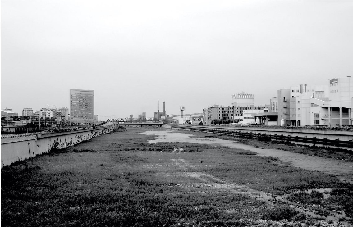
Fig.2. Torrente Polcevera. The river that crosses the valley is characterized by long periods of water shortage and heavy flows, associated with flooding risk.
