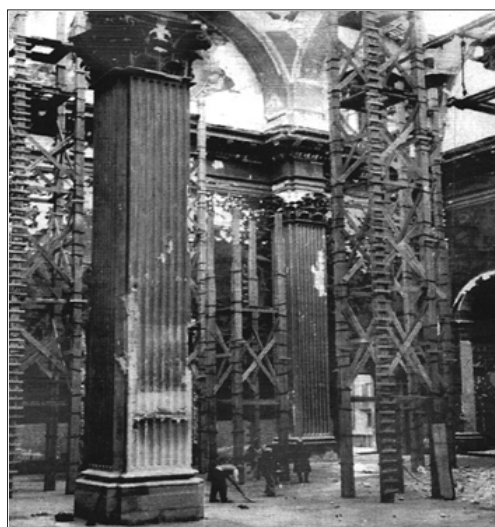
Figure 3: Interior of the cathedral during its inspection at the end of the war. We can appreciate the neo-classical columns inspired by the Pantheon in Paris and the remains of the Sert murals (archive: Manuel Gausa Raspall architect).
