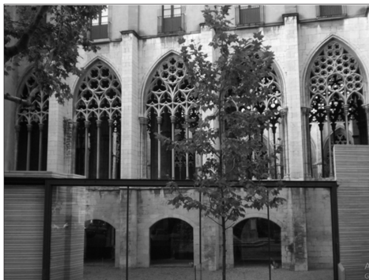
Figure 9: View of the Gothic cloister - with the Romanesque plinth - from the Meder river side banks walk.
