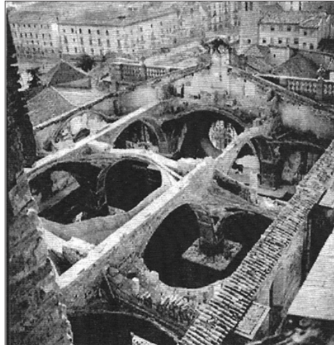
Figure 1: View of the remains of the cathedral roof after the bombing of 1939, shortly before the end of the war (archive: Manuel Gausa Raspall architect).
