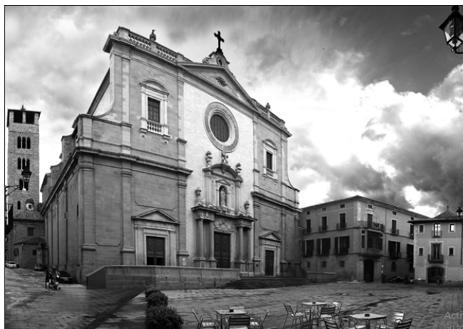
Figure 8: Main neo-classical facade of the cathedral, with the bell tower in the background and the access square.
