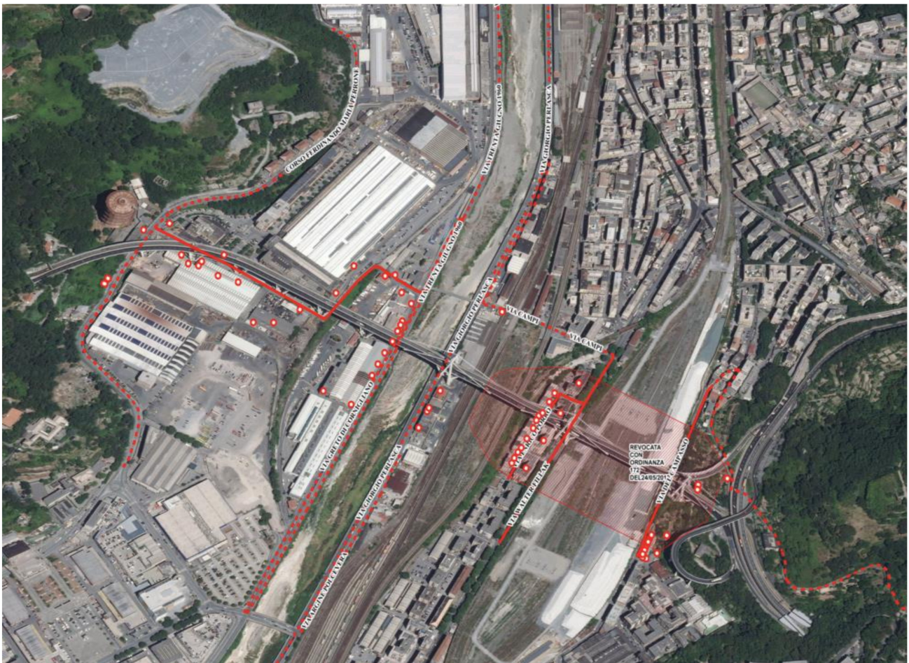
Figure 2. The ‘red zone’ that was totally blocked after the collapse. Red points are the residents and industrial owners without any vehicular accessibility to their properties. (source: http://www.commissario.ricostruzione.genova.it , accessed on 29 August 2020).
