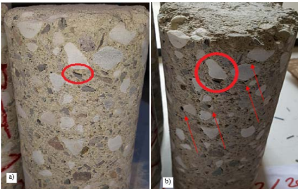
Figure 6. a) MIX 1 – w/c = 1.0: high porosity and water lenses on the surface of the aggregates. b) MIX 5 – w/c = 1.2: diffused porosity and water lenses on the surface of the aggregates.
