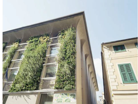
Fig. 6 INPS green façade, Genoa (Italy).
