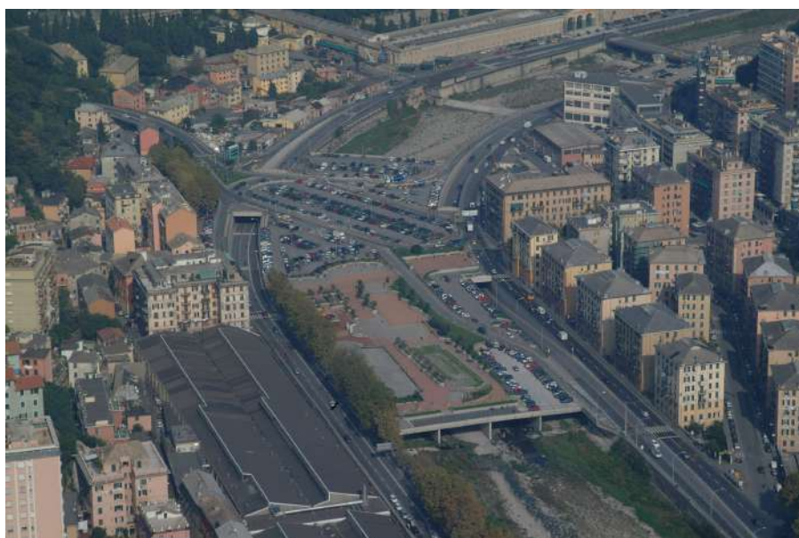
Figure 2 - Urbanisation in the valley floor and partial coverage of the Bisagno stream
