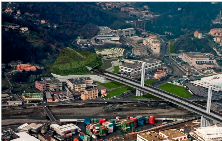
Figure 3. The new bridge on the Polcevera River. (Source: Autostrade per l’Italia S.p.A.).
