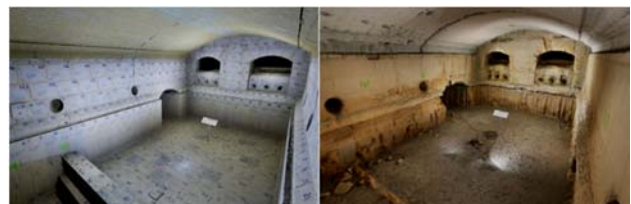
Fig.1. Glass furnace in new conditions (left) and before demolition (right)
