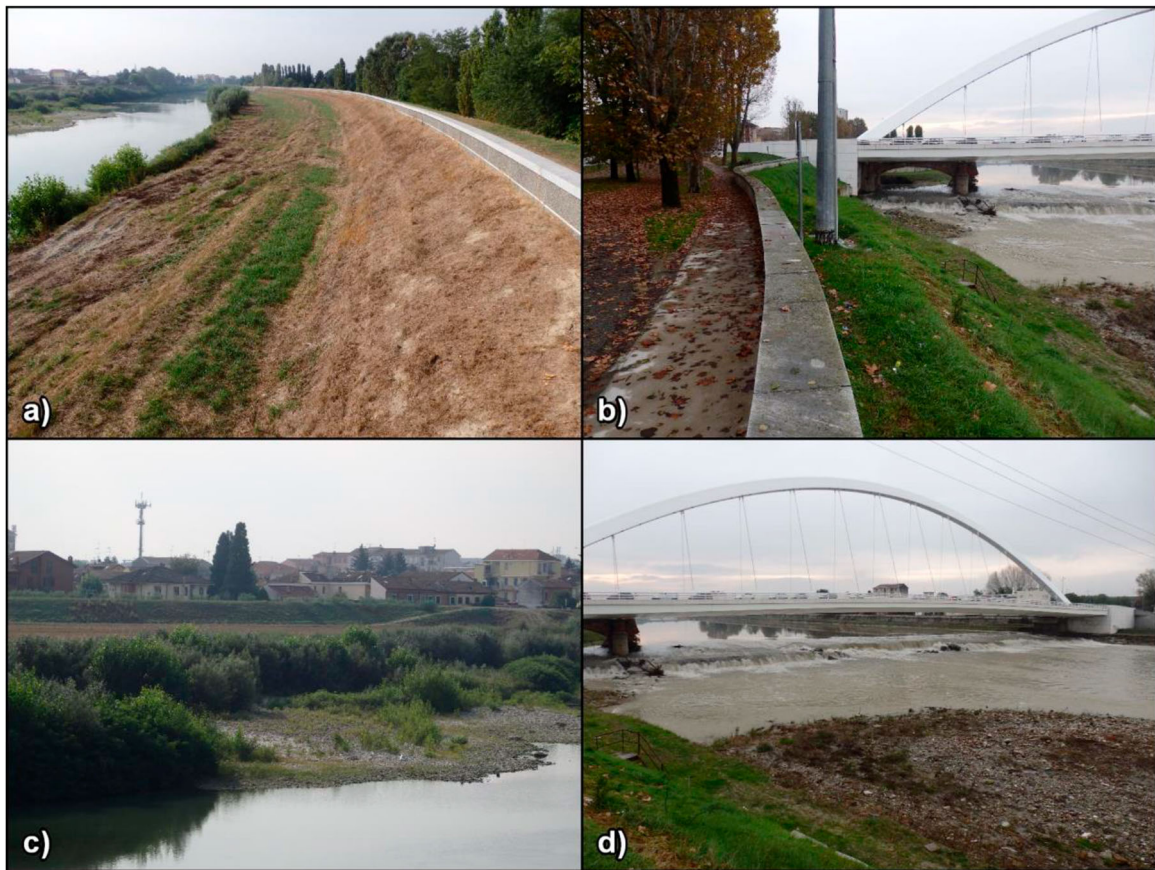
Figure 5. Different types of river-related anthropogenic structures along the Tanaro River urban stretch. (a) Trapezoidal cross-section levee with a concrete wall on top. (b) Concrete-wall levee. (c) Trapezoidal cross-section levee. (d) The Meyer Bridge and the consolidation check-dam representing the slab foundation of the demolished Cittadella Bridge. Photos by A. Mandarino.
