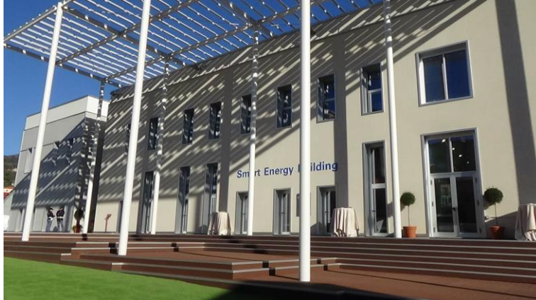
Figure 13: SEB building in Savona Campus
