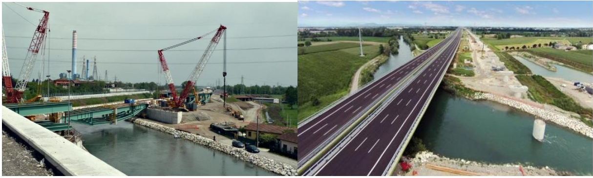
Figure 3: Muzza Bridge, (a) view during construction, (b) view in final configuration
