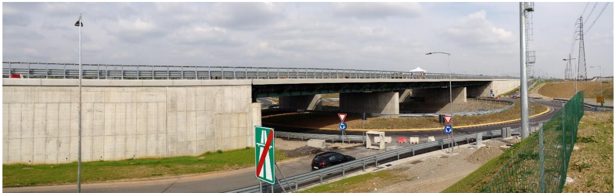
Figure 1: VX Bridge: view
