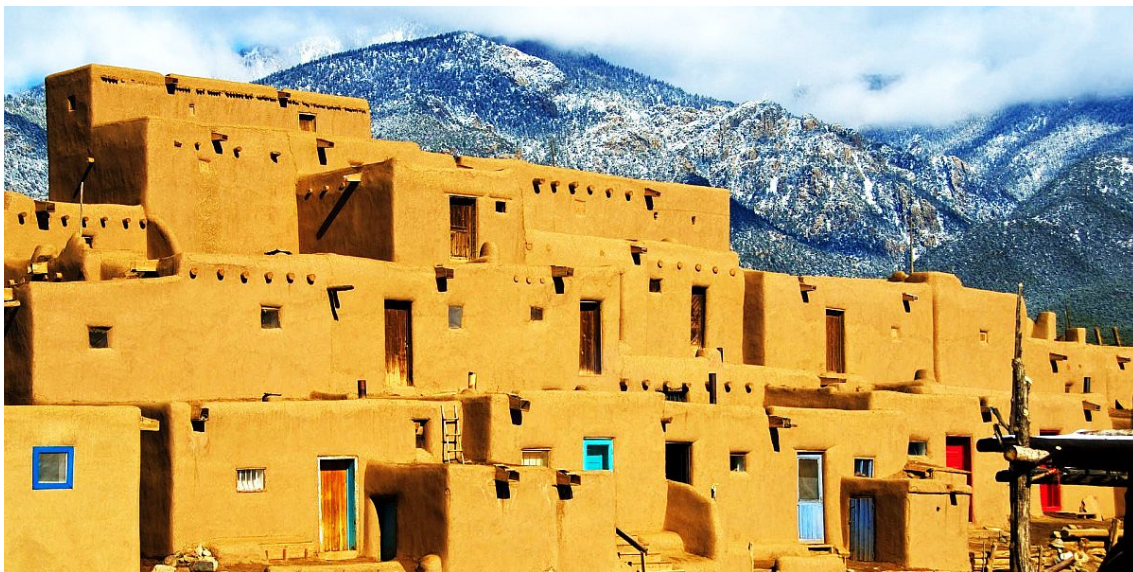
Figure 4. Ancient unstabilised adobe dwellings inhabited by a native American tribe of about 150 people at Taos Pueblo in New Mexico (USA).
