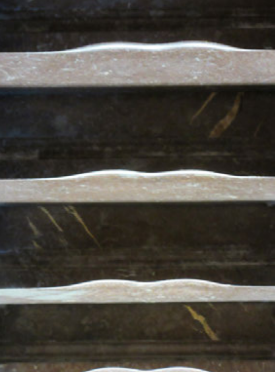
FIG. 1. The stairs to the relics of the Apostle Saint James (Cathedral of Santiago), consumed by the descending pilgrims' step.
