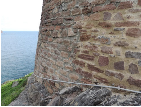
Fig. 5- Tower of Porto: the restored surface.
