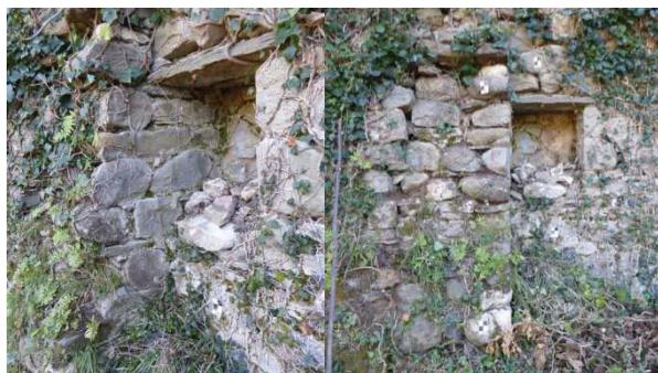
Fig. 07 : Wall H where - on the side of one of the niches - one can see a contemporary perpendicular wall, later cut
