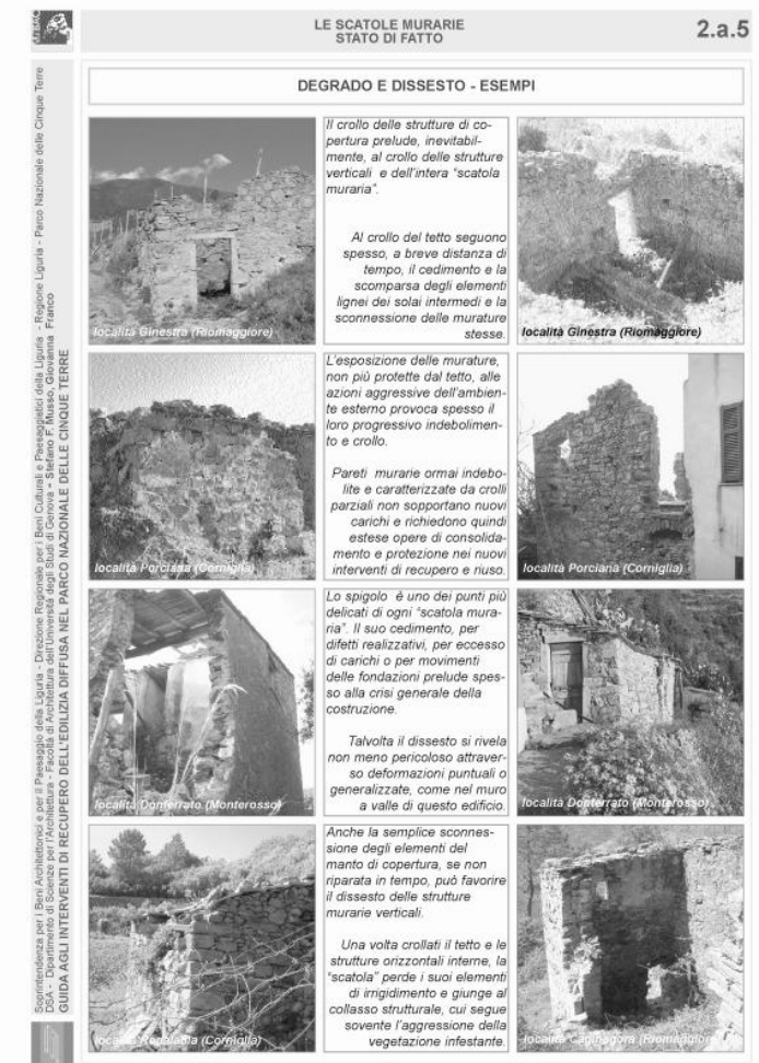
Figure 2. A inner page of the “Guida...” for the “Cinque Terre” National Park showing and explaining the recurrent problems of material decay and of structural instability that affect the traditional “masonry boxes” of the rural buildings of the Park.
