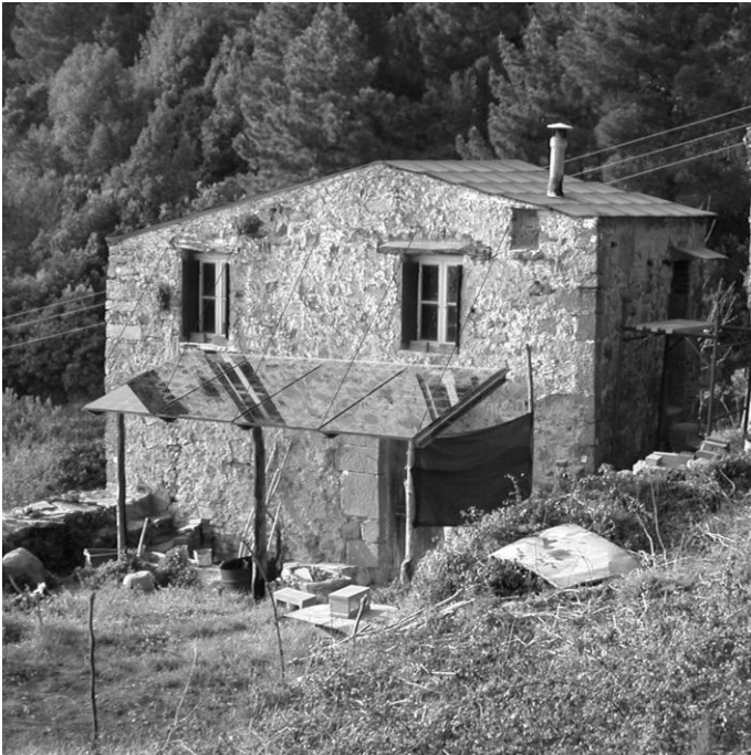
Figure 2. Photo-simulation on the same building of Figure 1. The plastic shelter has been substituted with a glass photovoltaic one for energy generation
