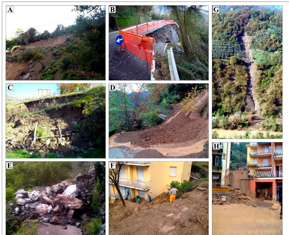
Figure 8. Examples of the different types of shallow landslides induced by rainfalls and the resulting damage: (A), roto-translational slide; (B), rotational slide downhill road cuttings, resulting in the partial collapse of the roadway; (C), shallow landslides on terraced slopes, with the collapse of the retaining walls; (D), complex movement uphill road cuttings, resulting in the roadway obstruction due to debris, blocks and vegetation; (E), rockfall; (F,H), soil slips and slow-moving earth flows, resulting in significant damage to buildings and man-made structures due to mud and debris; (G), rapid earth flow.
