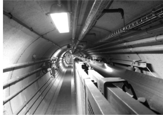
Figure 3: Underground conveyor belt inside a concrete-made mini tunnel, with safety equipments.
