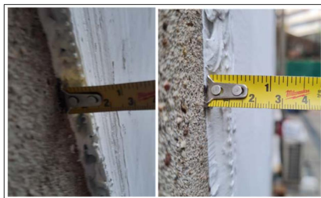
Figure 13. Total thickness of the nanotechnological mortar at the end of the laying.
