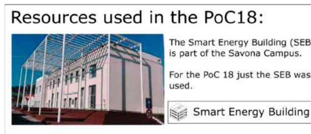
Figure 10. Smart Energy Building (SEB) in Savona Campus (Genoa University, Seville).
