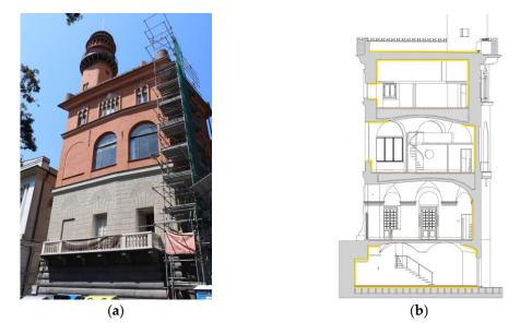
**Figure 8.** (a) The building after the restoration of the facades (Formento restauri). (b) A section of the building indicating the position of the insulation layers (in yellow).
