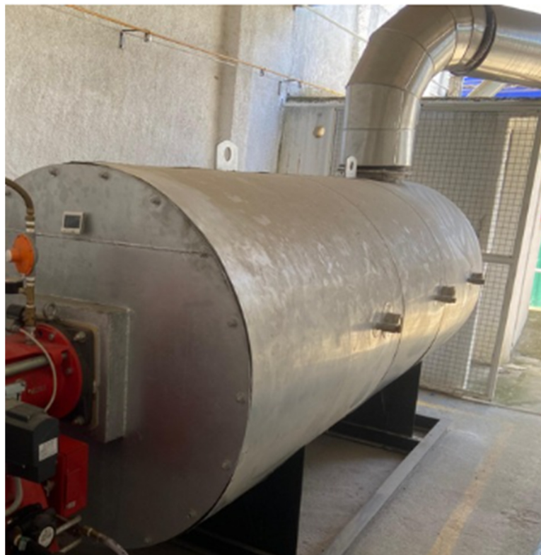
Figure 2. Hydrogen furnace at the Advanced Institute of Technology and Innovation, Recife, Brazil.
