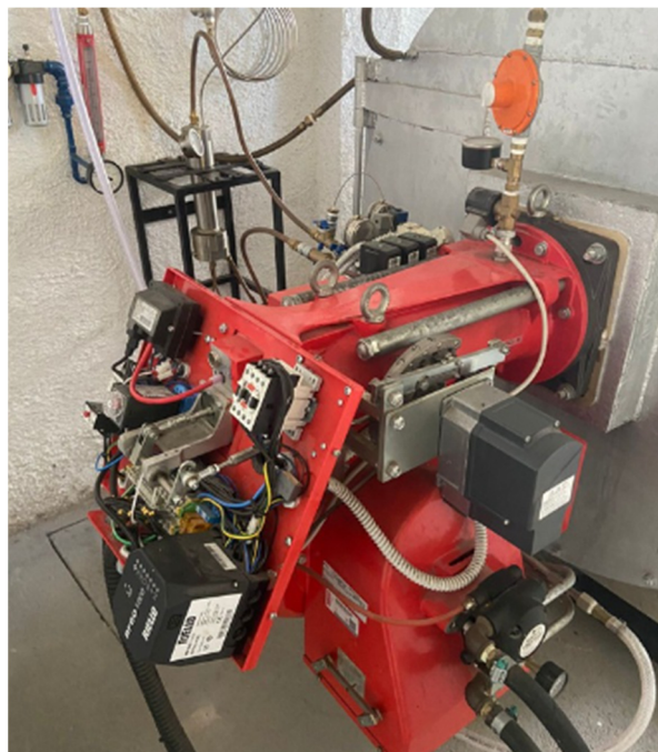
Figure 1. Hydrogen burner at the Advanced Institute of Technology and Innovation, Recife, Brazil.
