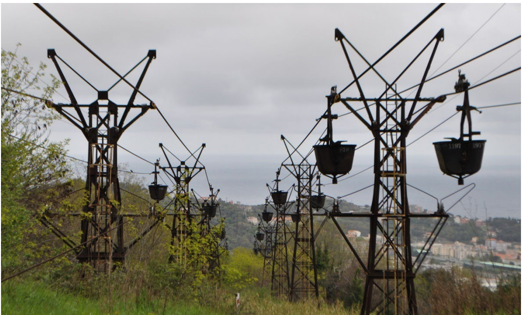
Figure 1: View of the Savona-S. Giuseppe Coal Cableway from one of the intermediate stations in Ciantagalletto, Savona, Liguria. Photo by F. Pompejano (©Land-In-Pro, 2023 - CC BY-NC 4.0).
