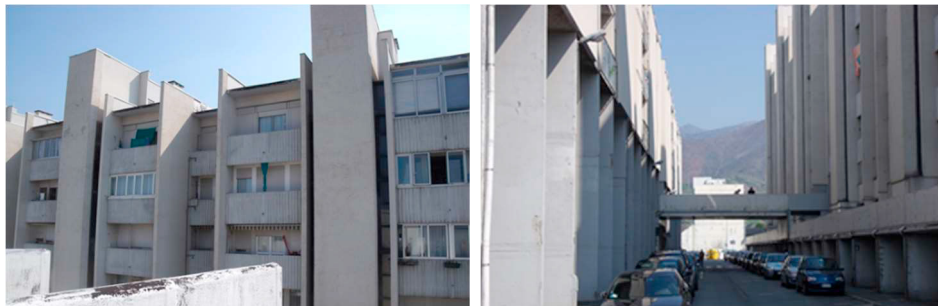
Fig. 7. Details of “Washing Machines”.
