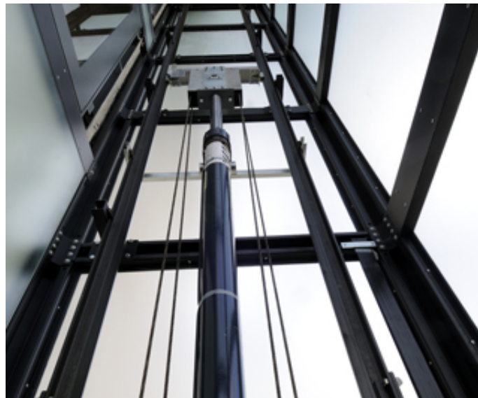
Figure 2.4: An example of roped hydraulic elevator - the cabin is moved along the shaft by pushing the ropes by the piston. The main pulley in this picture is hidden by a protection safety carter
